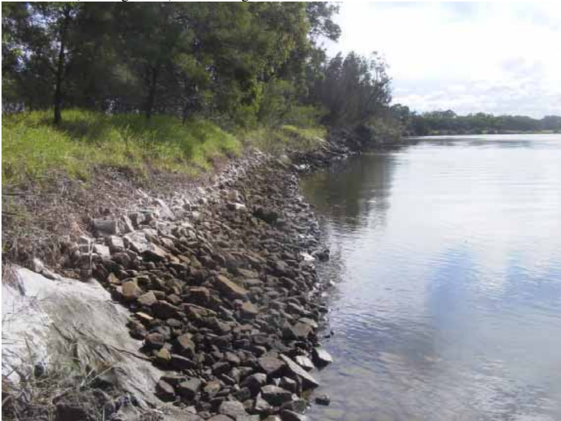
Figure 23 Engineered Rock Rubble embankment looking north of mangrove band with failed and slumped bank in foreground.
